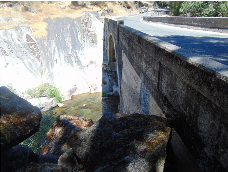
Photo 4. Camera facing south. Note exposed stacked masonry abutment
