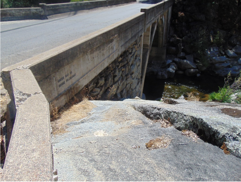
Photo 4. Camera facing south. Note exposed stacked masonry abutment
